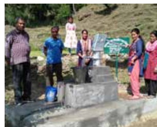
Completed handpump construction for SC Community in Pankot
